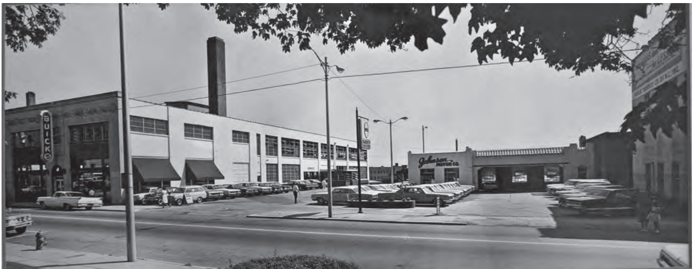
Figure 47: The Johnson Buick parking deck, 1968 (Courtesy Noell Nicholson Schepp)
