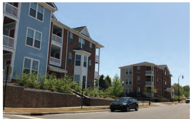
Figure 93: Southside Revitalization Phase II Buildings
