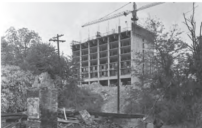
Figure 109: J.J.Henderson towers under construction, 1976 Source: Open Durham
