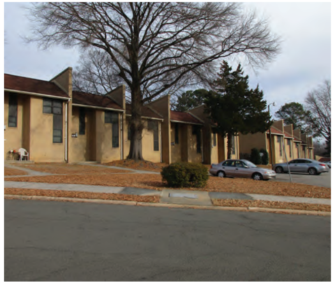
Figure 60: Existing Liberty Street Apartments
