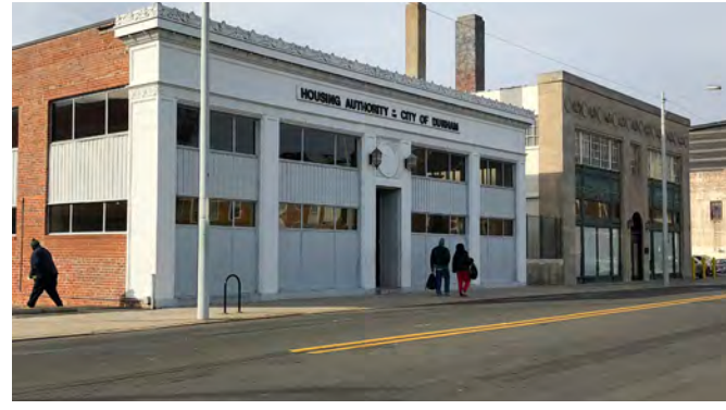
VIEW OF DHA OFFICE
