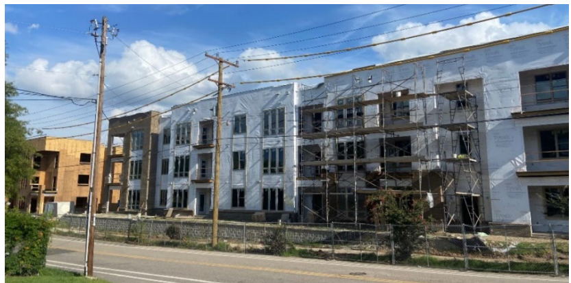
Construction of Elizabeth Street Apartments
